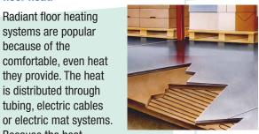
transfers directly from the floor to you rather than to the air in the room, you feel warm even though your thermostat is at a lower setting. When the tubing, cables or mat system are submerged in sand, they can qualify for lower load management electric rates because heat can be stored. If the area utilizing radiant floor heating does not allow for the application of heat storage, a backup heat source is necessary to gualify for load management electric rates.
